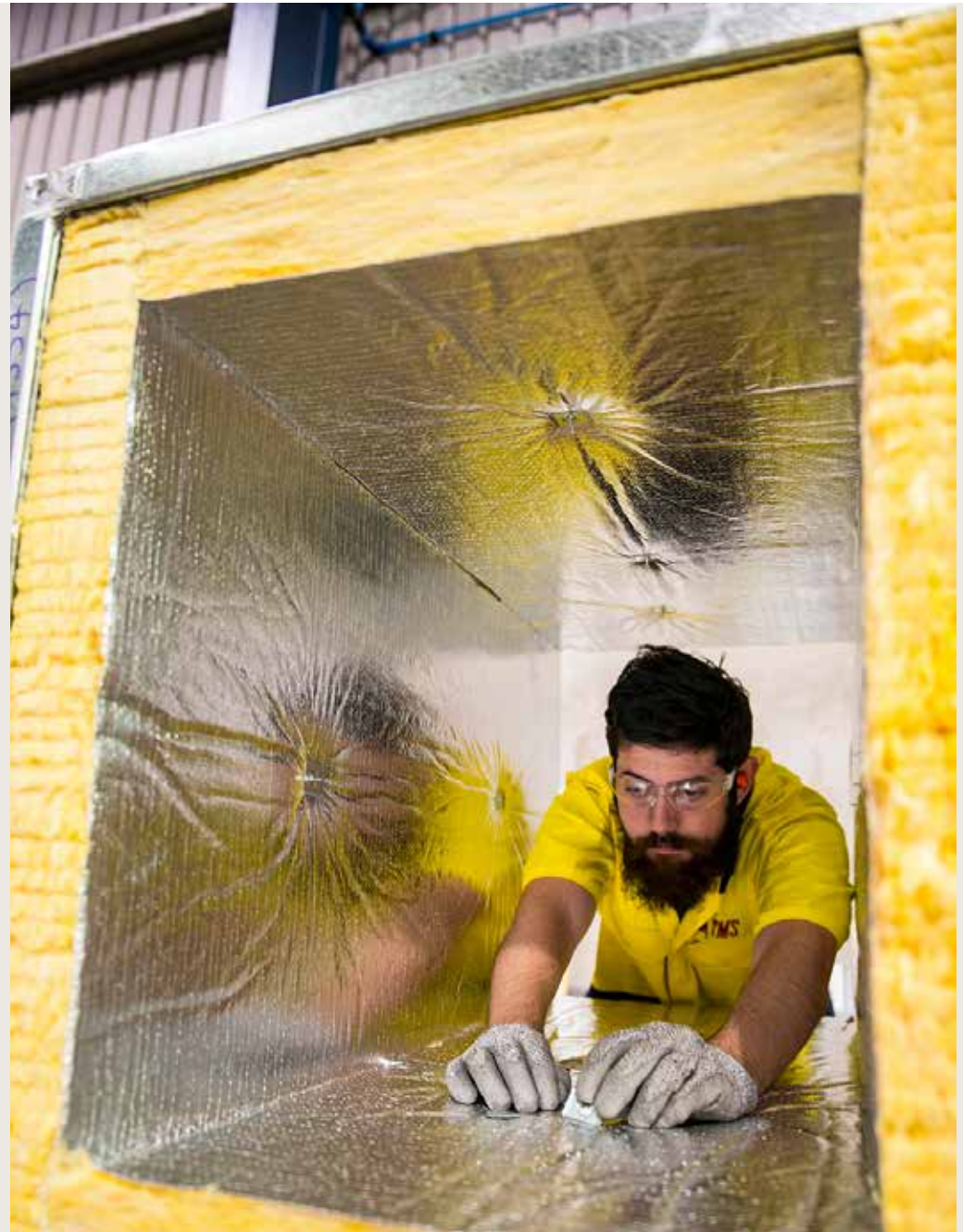
INSTALLATION OF THE BRADFORD SUPERTEL INSULATED HVAC DUCT
