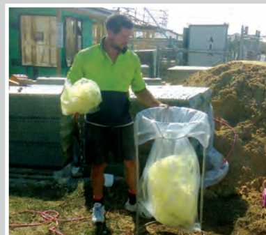
Monier packaging waste reduction project in Victoria
